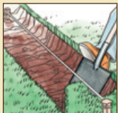
1. Stake Out/Remove Sod
