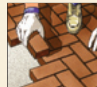
5. Lay Paving Stones
