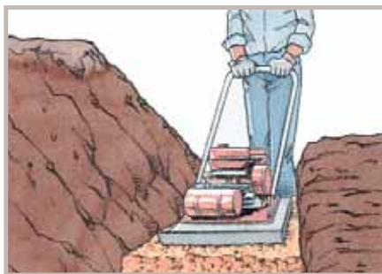
LEVELING PAD COMPACTION
